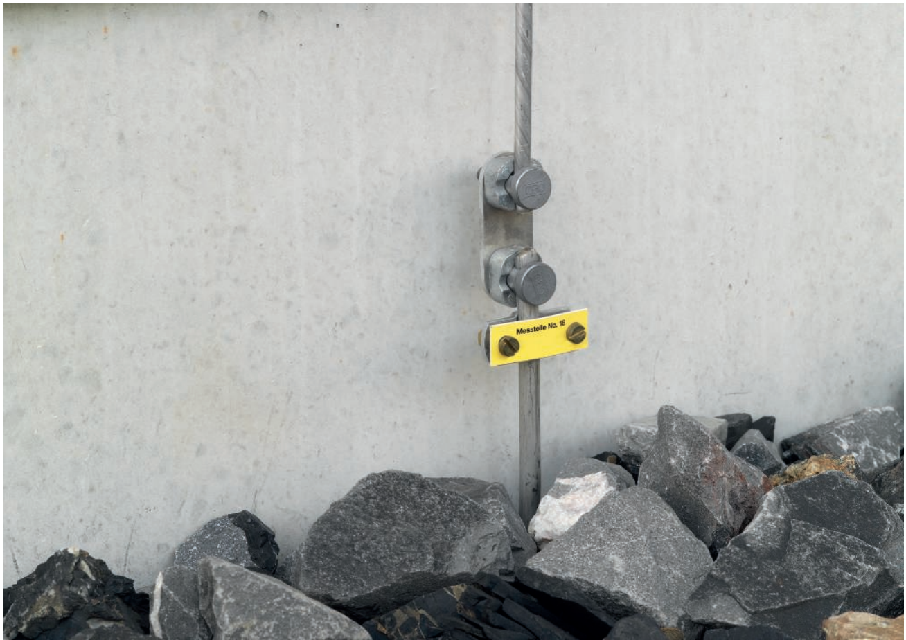
Separation point on a metal facade
