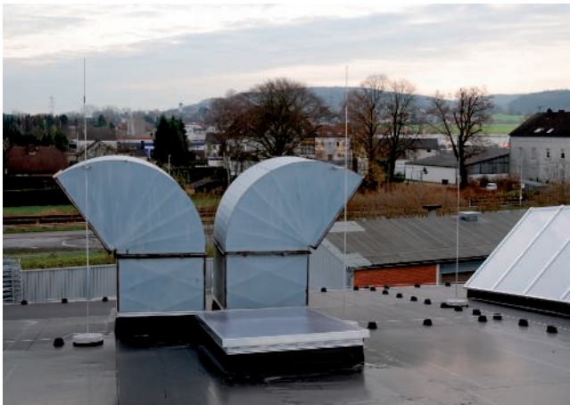
Isolated system with GRP holders
