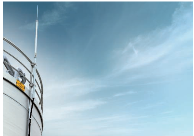
Isolated lightning protection with isCon®
