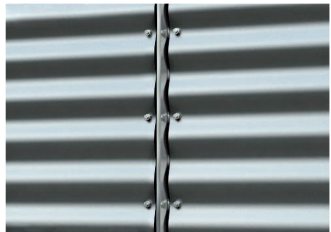
Example: use of horizontally connected facade elements as an down-conductor system
