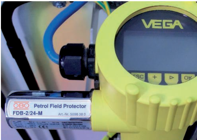
Sensor with Petrol Field Protector FDB
