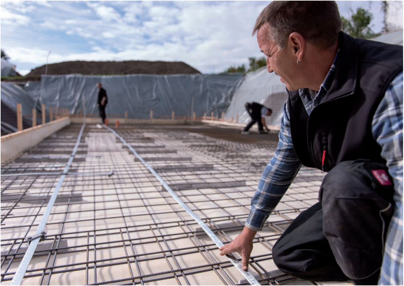
Installing a foundation earth electrode
