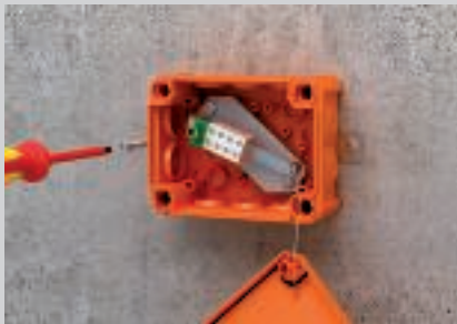
Quick lid mounting through 90° rotation of the corner screws.
