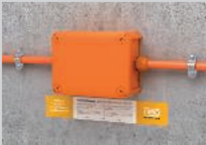
Fully installed FireBox with identification plate.
