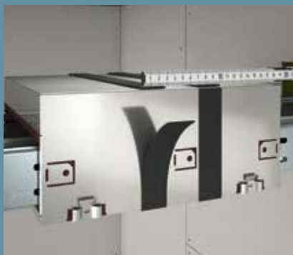
Measure the wall thickness and apply the graphite strips at the appropriate distance
