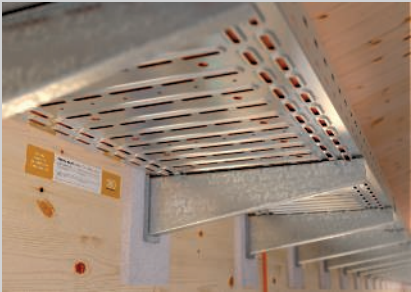
Bracket mounting on the side of the wooden beam with rear fire protection plate.
