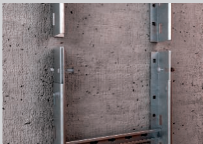
Joint connection with screwed-on connector.
